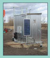
The Bear Solar Electric **Control System** offers zero emission technology for replacing pneumatic control devices at well sites using methane fuel gas in nearly every situation, contributing to the reduction of methane emissions in the atmosphere.
